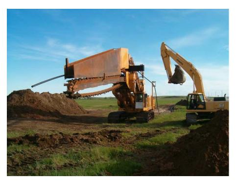
Figure 4.2 Slotted HDPE Pipe Threaded Through a Continuous One-Pass Trencher Prior to Installation, Ellsworth AFB, South Dakota
