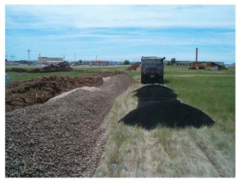
Figure 4.1 Stockpiling of Biowall Materials Prior to Mixing at the BG-05 Site, Ellsworth AFB, South Dakota (from left to right is mulch, sand, gravel, and magnetite ore)
