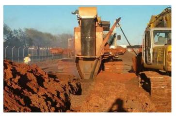
Figure 1.1 Installation of a Permeable Mulch Biowall at Altus AFB, Oklahoma
