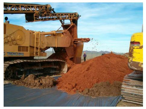
Figure 5.2 Laying Excavated Trench Soil on Plastic Sheeting, Altus AFB, Oklahoma
