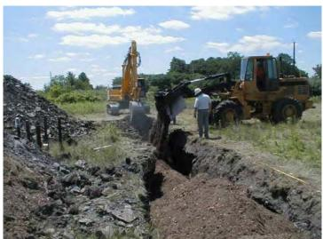
Figure 3. Installation of the Ash Landfill Biowalls
