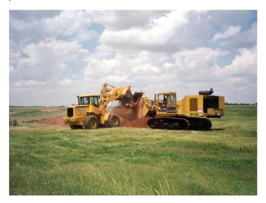
Figure 3. LF-03 Biowall Installation Using a Continuous One-pass Trencher
