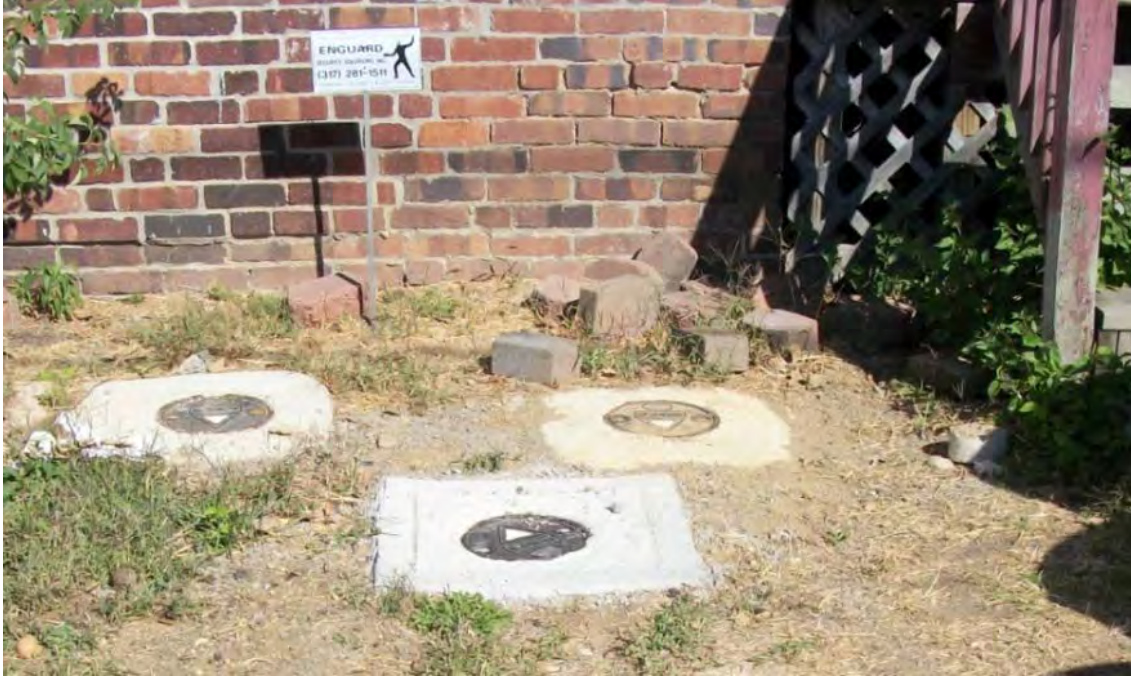
Figure 3-17. Nested monitoring well 1 and SGP1 are located immediately south of the 422 side front wall. SGP1-16.5 and MW-1A is by the wall, to the left of the sign. SGP1-9 and 1-13 as well as MW-1C are by the wall, to the right of the sign (next to the pile of bricks). SGP1-3.5 and 1-6, and MW-1B are in the installation visible in the center foreground.
