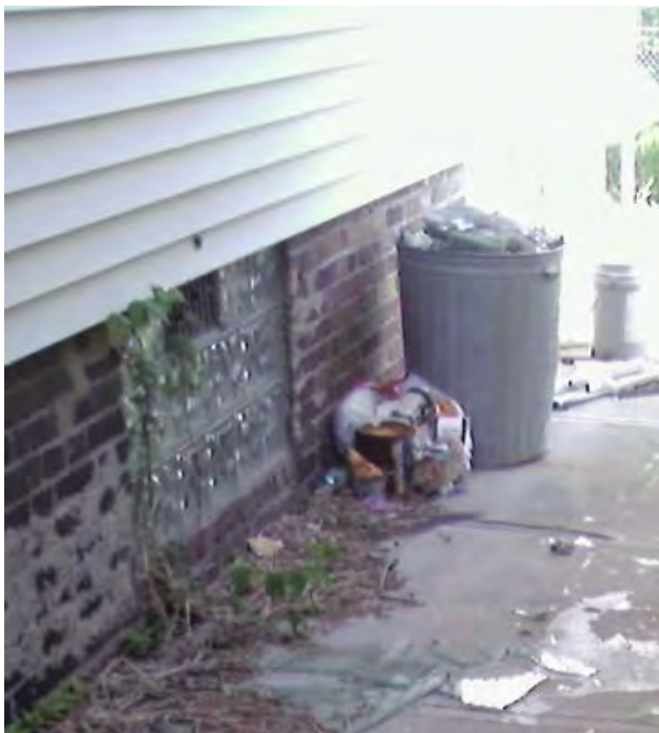
Figure 12-6. Note height of basement window and vent (sealed for this study).
