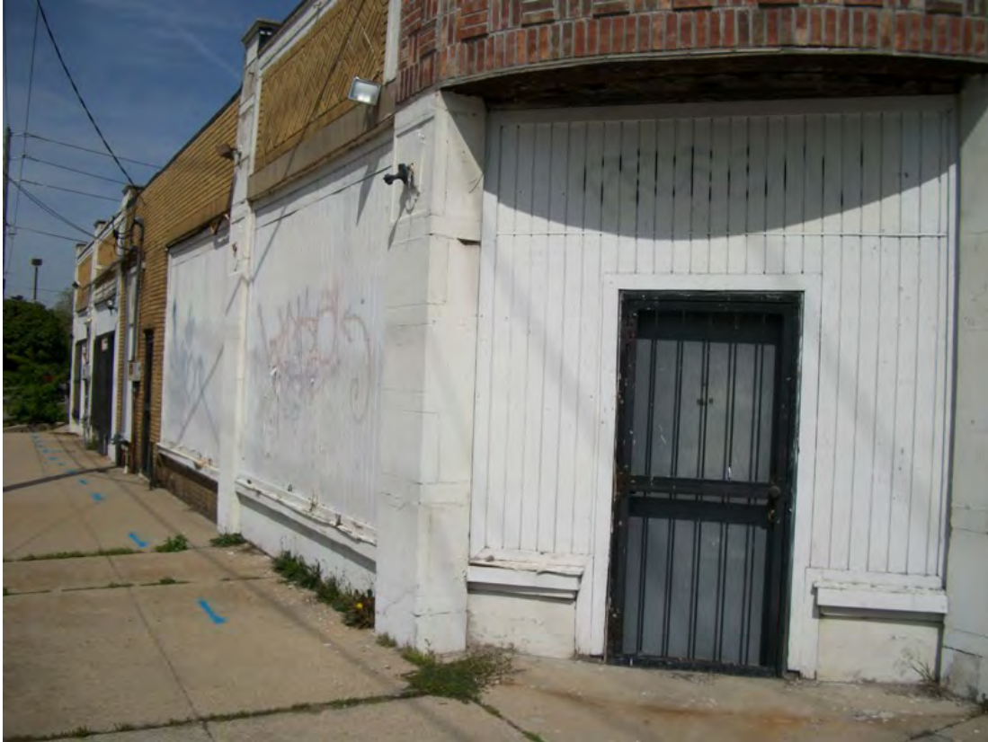
Figure 3-5. Looking toward southeast corner of adjacent commercial quadruplex.
