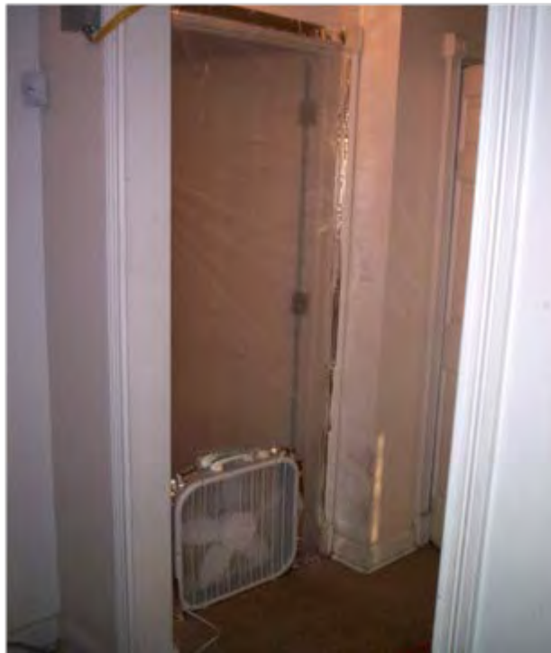
Figure 12-2. Fan position in stairwell (note plastic sheet over doorway).
