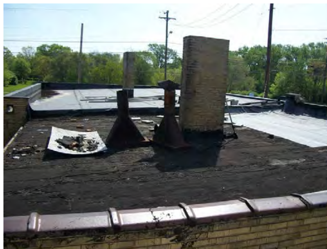
Figure 3-4. Roof of adjacent commercial quadraplex.
