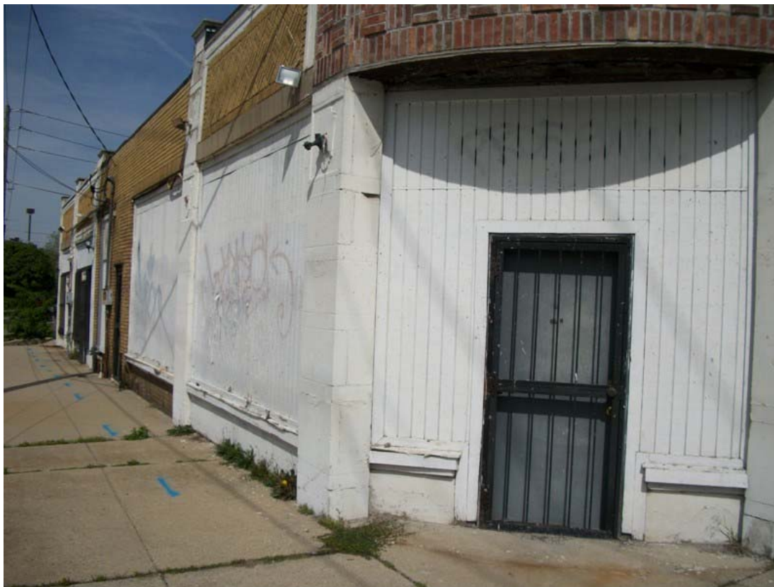
Figure 3-5. Looking toward southeast corner of adjacent commercial quadraplex.
