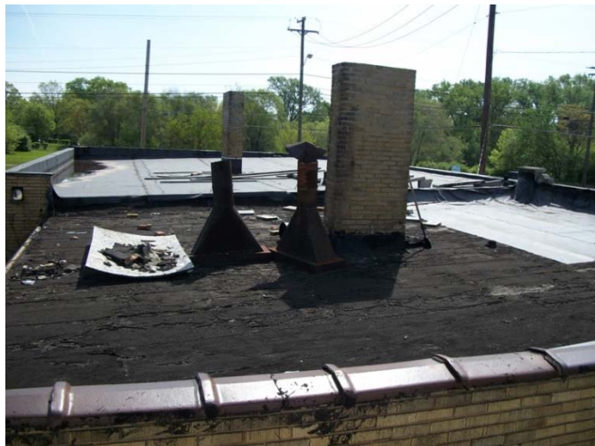
Figure 3-4. Roof of adjacent commercial quadraplex.
