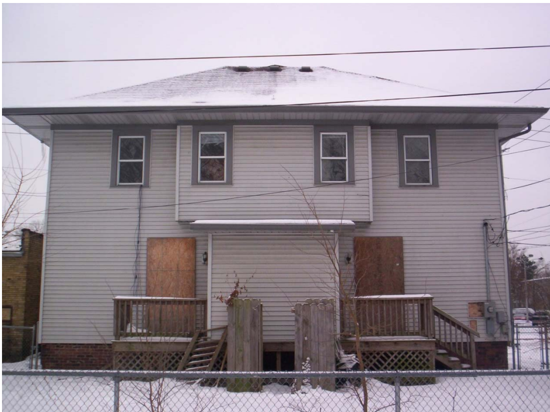
Figure 3-9. 422 (left) and 420 East 28th Street in January 2011.
