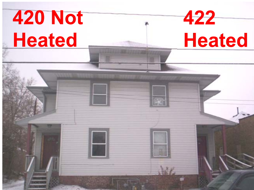
Figure 3-8. Front view of duplex under winter conditions showing designation of sides and HVAC setup.
